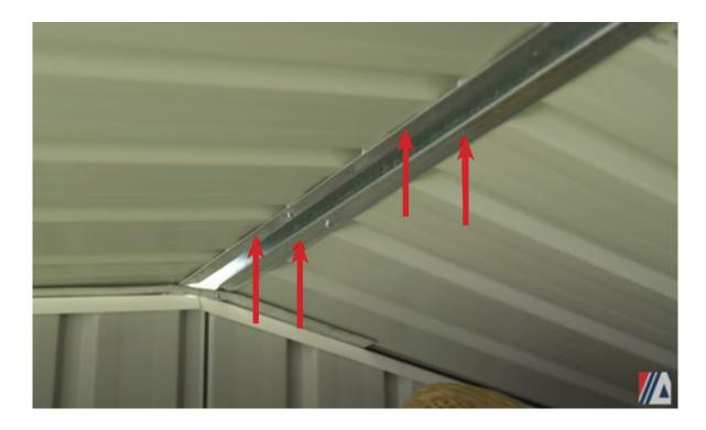
THESE POSITIONS DO NOT HAVE PRE-PUNCHED HOLES SO USE THE SUPPLIED DRILL BIT TO PREDRILL HOLES THROUGH THE RIDGE BEAM, THE ROOF PANEL CHANNEL INSIDE IT AND THE ROOF SHEET.
