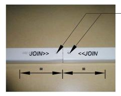
Finished Channel. The joined channels should now look like the picture with the CSJ positioned equally inside of the joined channels. Drill out holes with 1/8" drill bit in CSJ to match the holes in channel. Drilling of screws on the joined channels is being done after sheets are locked on the spliced channels.
