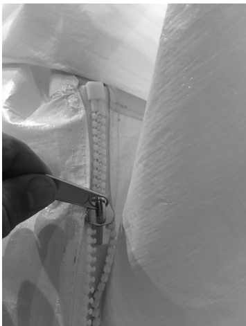
Step 20) Zipper walls together in downward motion.
