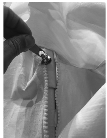
Step 19) Join zipper at the top of the walls.
