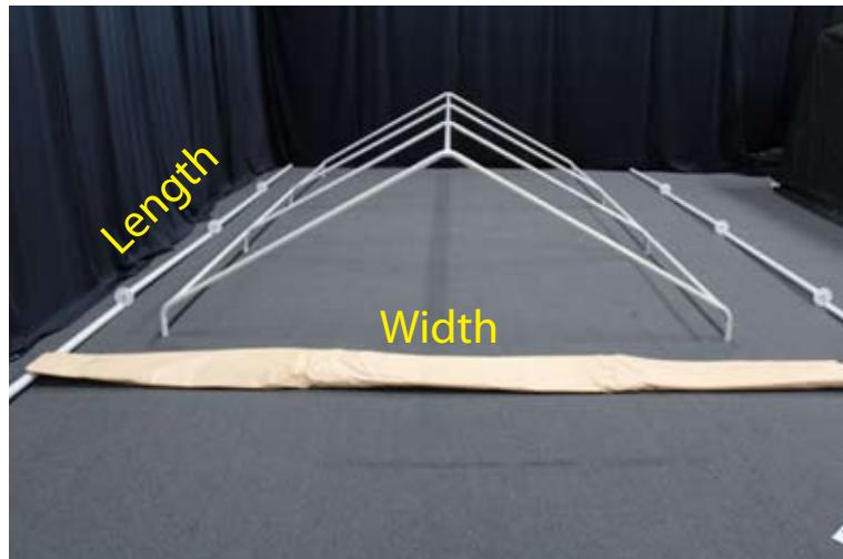
**1)** Now that the roof frame work is complete, you can begin to attach the fitted cover. Start by laying out the cover to determine which way it is folded, the length or width of the frame.
