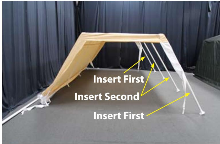
**9)** Begin to attach the legs to the frame. Place each leg next to the three and four way fittings. Starting with the two outside legs grab the base of the 3-way corner fitting. Lift the frame and insert the Leg into the 3-Way fitting. Next insert the center legs.
