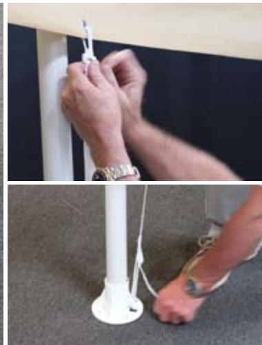
**11)** Pull down and attach the leg skirt straps to the foot pads at each corner. Next attach the valance straps by clipping the plastic hook to the open grommet hole located on the cover's valance (4 total). Hook the plastic ring around the foot pad and tighten.
