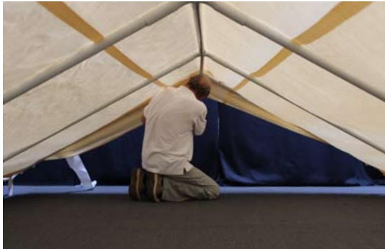
**6)** Continue attaching straps from left to right in a zig zag pattern starting at the two center peaks.
