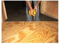
Drill 5/16" hole for the barrel bolt.
