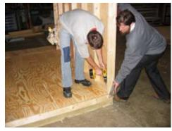
Now locate the first wall panel and set in place, make sure the wall is flush with the edge of the floor structure using an angle. Apply pressure from the outside and fasten with 2 1/2" screws.
