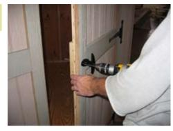
Next install and fasten the latch with 1 1/4" black head screws as shown.
