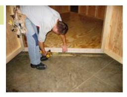
Place the small piece of duratemp siding (this is the piece we set aside to use underneath of the door) below the door opening and use the angle to make flush. Fasten with 1 1/4" screws, approximately 8" on center.
