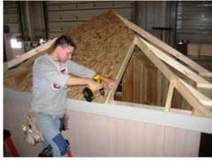
Fasten with 1 1/4" screws at each corner as shown, bottom corners first.
