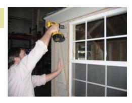
Install the shutters as shown and fasten with 2 1/2" screws.
