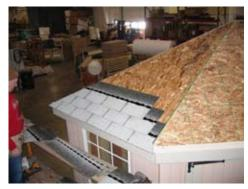
Continue attaching shingles to the top roof section, staggering as shown.
