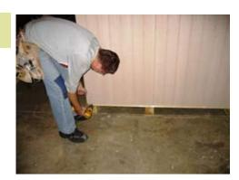
Fasten around the bottom with 1 1/4" screws every 8" on center.
