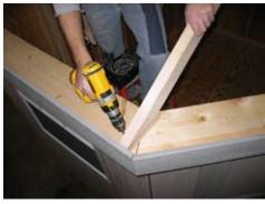
Next install the rafters as shown and fasten with 2 1/2" screws as shown.
