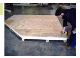
Set each sheet in place and make sure the sheeting is flush on both sides. Secure in place by driving the 1 1/4" screws through the sheeting into the 2x4's every 8".
