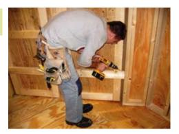
On the inside of the doors you will find a 2x4 brace. Remove the brace and set aside. You will use it again to help brace.
