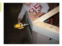
You will need 1 screw on each side and 1 from the outside through the trim into the truss.
