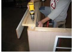
Install the top plate. Use the angle and make flush on the inside.
