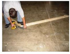
Fasten the first set of rafters at the peak with 2 1/2" screws as shown.
