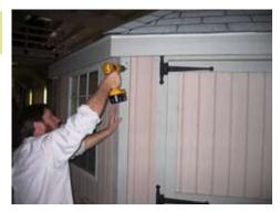
Now install the outside corners as shown and fasten with 1 1/4" screws.
