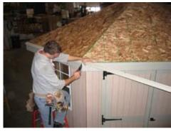
Use tin snips and cut at the corner as shown to fit
