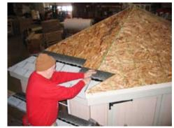
Use a utility knife and cut shingles at the ridge line as shown.
