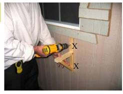
Next install the bracket for the flower box and fasten with 2 1/2" screws where shown.
