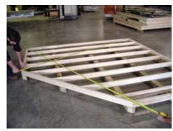
Place the 2x4's 16" on center on top of the 4x4 runners. Measure from corner to corner to square up.
