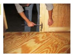
Hold the door in place and use hammer to tap on barrel bolt so it makes a mark for where to drill the hole.
