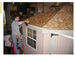
Next install the drip edge as shown. Fasten with  $1 \frac{1}{2}$  screws.
