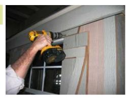
Install the trim at the top of the window and fasten with 1 1/4" screws.
