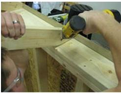
Insert screw on angle as shown to secure truss.
