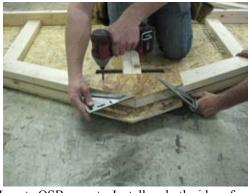
Locate OSB gussets. Install on both sides of peak. Secure with 1 1/8" zinc screws.
