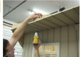
Secure with 2 1/2" screw from underneath overhang. First make sure rafter is in place.
