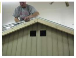
Drip edge goes around the edge of the roof as shown. You need to cut at the peak and also cut off at correct length.
