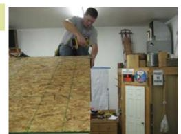
Insert 1 1/4" zinc screws through OSB sheeting into rakes.
