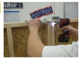
Secure top end with 2 1/2" screws as shown.
