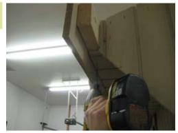
2x4 fascia will rest on overhang as shown. Secure going up through LP siding with 1 1/4" zinc screw.
