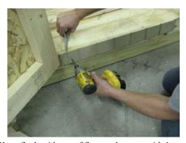
Keep flush with top of floor and secure with 1 1/4" screw.
