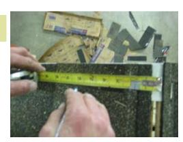
Measure 6" from the center of the peak as shown. Do this on each end at the peak.
