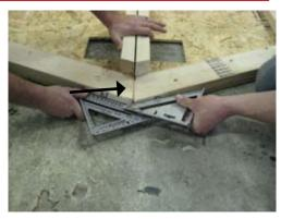
Before installing the gables, butt the ends together as shown. Make sure peaks meet at the point.
