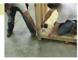
Make sure wall is flush as shown. Secure wall to floor with 2 1/2" screws.
