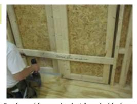
Continue with removing 2x4 from double door as shown.
