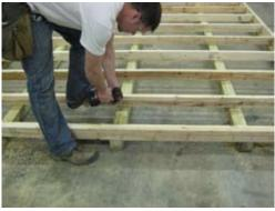
Once floor is square, secure each joist by using a 2 1/2" screw as shown.
