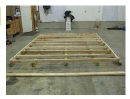
Once 4x4's are layed out, install 2x4 joist on top as shown. The 2x4's are 16" on center.
