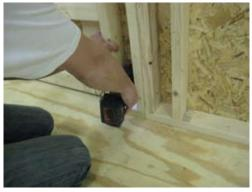
Secure walls with 2 1/2" screws as shown.
