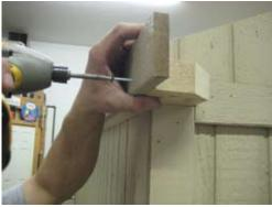
Insert 1 1/4" zinc screw from fascia trim into rake block as shown.
