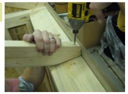
Once truss is in place secure with 2 1/2" screw.
