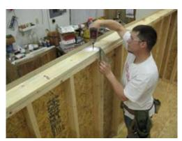
Make sure top plate is flush on inside wall.
