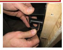
Use allen wrench to secure D-handle as shown.
