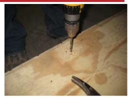
Use 3/16" drill bit and drill a hole where the barrel bolt made a mark on the floor. When closing the door, barrel bolt will insert in hole to keep door closed.
