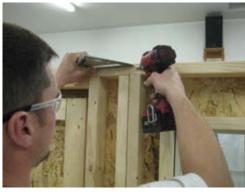
Once bottom is secured, make sure top end is flush as shown and secure with  $2 \frac{1}{2}$  screws.
