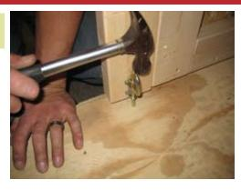
Now locate the barrel bolt located on the double door. Make sure door is closed and use hammer to tap on barrel bolt. This will leave a mark on the floor.
