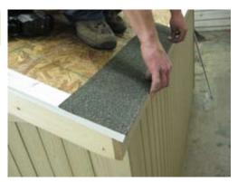
Shingles are provided by the customer. Begin by installing the starter strips as shown. Secure with 7/8" roof nails.
