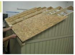
Next install roof sheeting. See roof layout for proper roof sheeting placing.
