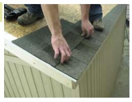
Install shingles as shown and secure with 7/8" roofing nails.
