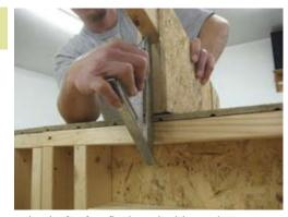
Keep heel of rafter flush on inside as shown.
