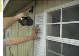
Make sure shutter is evenly spaced up and down with window and secure with white head screws provided for shutters.
