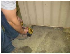
Insert 1 1/4" zinc screw every 8" to 10" on bottom edge of siding all the way around the building.
