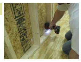
Secure back wall with 2 1/2" screws.
