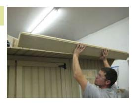
When installing fascia make sure 2x4 is up and trim overhang is down.
