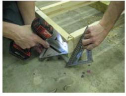
Next make sure joist and rim are flush with 4x4 runner and secure with  $2\ 1/2$ " screws.
