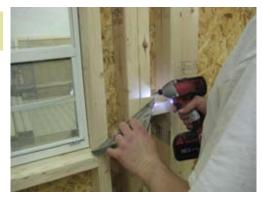
Secure wall splices with 2 1/2" screws.
