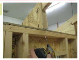
To complete truss in front secure with another 2 1/2" screw from inside as shown.
