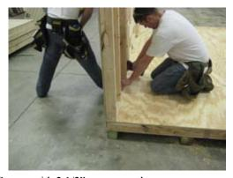
Secure with 2 1/2" screws as shown.
