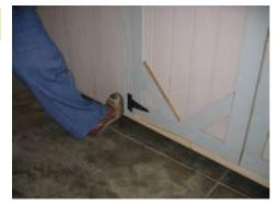
Use your foot to push in the door panel, so the siding is against the floor.
