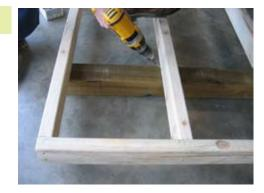
Once the floor is squared you can fasten the rest of the joists to the 4x4's.
