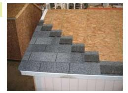
Cut ridge cap in the shape shown in picture and start to place the cap on the top of the building.
