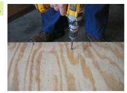
Use a 5/16 drill bit and make a hole for the barrel bolt to slide into.
