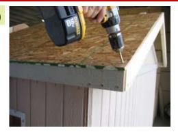
Measure and then fasten at the top once trusses are in the correct position.
