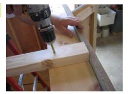
Install the truss as shown. The trusses for the larger building will need to be assembled.
