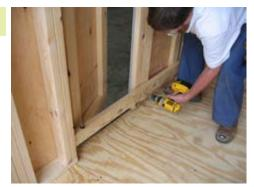
Before installing last wall, remove door packaging piece as shown.
