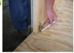
Hold the door against floor and make a mark around the barrel bolt as shown.
