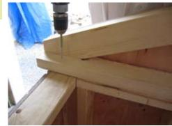
Once you have this positioned, fasten. Repeat this on the other side. If you can not obtain a 5 1/2" reading on either side split the difference between the two.
