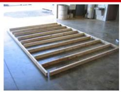
Layout the parts for the floor as shown. Refer to the diagram for spacing. We will assemble an 8x12 workshop in this manual. The other sizes are the same basic structure, just larger.
