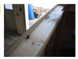
Use the door packing brace and fasten the wall braces together as shown.
