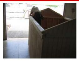
Note how the 2x6 will look. Note the markings on it are to show the placement of the trusses.
