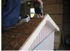
Once the bottom sheets are installed, install top sheets. Different sizes may have varying size sheets. The diagram will show the size and layout.
