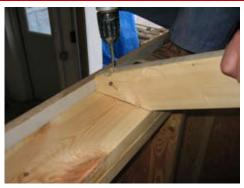
Fasten tursses from the outside, underneath the 2x6 and into the truss. Use one 2 1/2" screw on either side of the splice, if truss rests on splice.
