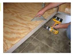
Install siding strip beneath door. Be sure to keep even with the floor as shown with the square.
