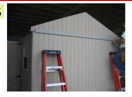
Position gable on top of wall as shown. The larger sizes will have to be assembled first before installing.
