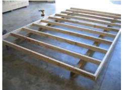
Once the frame is fastened lay the 4x4's underneath. Refer to the layout diagram for number of 4x4's and spacing. On the larger sizes you will need to splice the 4x4's by applying a gusset to the side of them.
