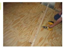
Install the wall brace. Position it beside the center truss marks. This will hold the building together and provide strength.
