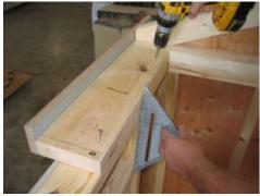
Install first piece of 2x6 with trim fastened to it. Keep trim face up as shwon. Match sets for each side of the building. Keep inside even as shown with square. Fasten into bottom wall.
