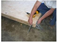
Place the piece of plywood on top of the joists. Make sure that the plywood is even with the joists as shown.
