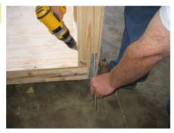
Make sure the edge is even with the floor, and the siding is in against the floor. You can push in the siding against the floor with your shoe.
