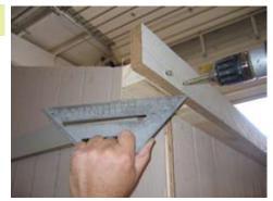
Fasten rake together as shown. Keep even on top and screw together.
