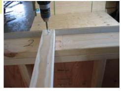
Install the other side of the gable. You may need to pull or push the wall in order to obtain the correct position before fastening.
