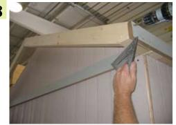
Fasten first piece of OSB per diagram layout. Only fasten at the bottom to begin with. Before fastening the top you will need to make sure all the measurements are correct. (make sure trusses are not leaning to one side or the other).
