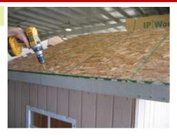
You can use 1 1/4" screws to fasten. Fasten on the bottom outside edge.
