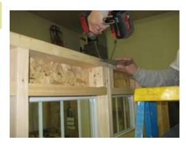
Make sure the walls are flush on the inside and secure with 2 1/2" screws as shown.
