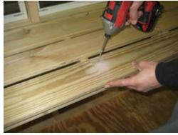
Secure with 1 1/4" screws , where needed on top.
