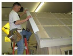
Install rake cover with wider side on top.
