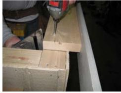
Next install top plate, make sure 2x6 is at the pencil mark as shown on last picture.
