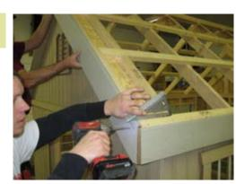
Make sure it is flush on the top of the purlins and secure with 2 1/2" screws.
