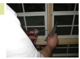
Use 1 1/4" screws to secure wall as shown.
