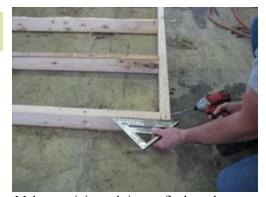
Make sure joist and rim are flush as shown and secure with 2 1/2" screws.
