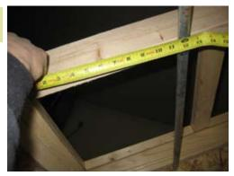
Measure 12" from top plate to where pipe should be fastened.
