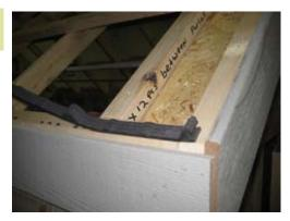
Install rubber closures on bottom edge as shown.
