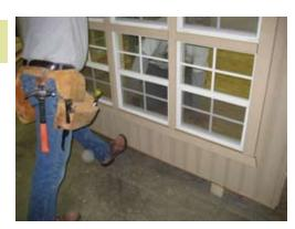
Apply pressure on all walls as shown before securing with 2 1/2" screws.
