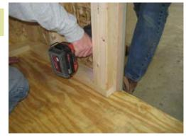
secure wall with 2 1/2" screws.
