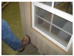
Apply pressure on outside while fastening with 2 1/2" screw from inside as shown.
