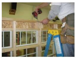
Next make sure walls are flush on inside and secure with 2 1/2" screw.
