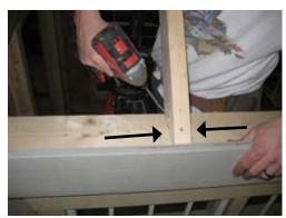
When securing truss use (3) 2 1/2" screws as shown (1) on top and (1) on each side of the truss.
