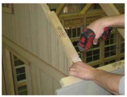
Install 2x2 Bird Block on top of gable as shown, and secure with (2) 2 1/2" screws.
