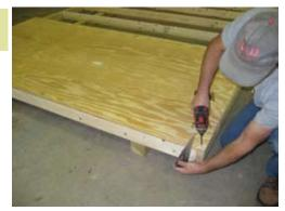
Set sheeting in place using angles to ensure sheeting is flush on both sides. Secure in place by driving 1 1/4" screws through the sheeting and into the 2x4's every 8".
