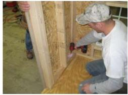
Apply pressure on outside and secure with 2 1/2" screw.
