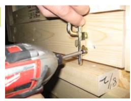
Next install barrel bolt on inside top door and secure with 1 1/4" screw.
