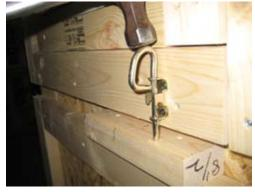
Push barrel bolt down and tap on with hammer to locate where to drill 5/16" hole.
