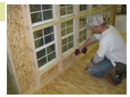
Apply pressure on the outside as before and secure with 2 1/2" screw.
