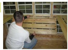
After both sides are installed, install center shelf and secure with 2 1/2" screws.
