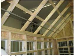
Install C-clamp on every truss.
