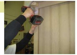
Secure with 1 1/4" screws as needed on all 4 corners.
