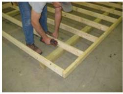
Next measure 16" On Center, and secure 2x4's into 4x4 by toe nailing a 2 1/2" screw on both sides
