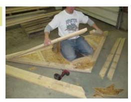
Next locate gable wall and use it for truss assemble as shown.
