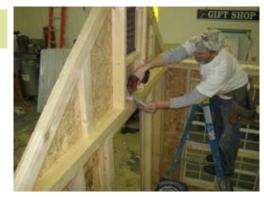
Make sure 2x4's are flush and secure with 2 1/2" screw as shown.
