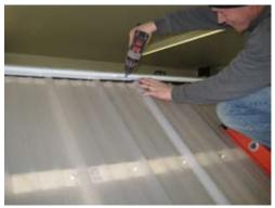
Continue with inserting 2" screws.
