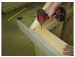
Secure with 2 1/2" screws once gable is in place.
