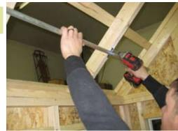
Use 1 1/4" screws to secure pipe in place.
