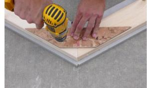
Set truss Gusset in place and fasten with (8) 1 1/4" black headed screws.
