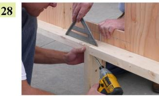
A gable with transom windows: Bring the two section together and secure with 2 1/2" screws, toe nailing.
