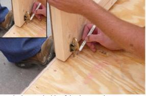
On the bottom inside of the door, apply pressure on door and mark with a pencil to drill 5/6" hole for barrel bolt.
