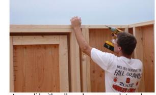
As you did with wall panels, use an angle to make sure 2x4's are flush and fasten with 2 1/2'' screw.
