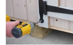
Fasten the bottom door hinges with 2 1/4" black headed screws.
