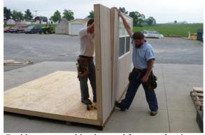
Position next panel in place and fasten to sheeting along the bottom with 2 1/2" screws...
