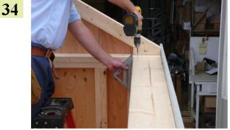
Next find the 2x8 plate, now lay the 2x8 plate making it flush with the 2x4 on the inside of the wall. Fasten the 2x8 to the 2x4 with a 2 1/2" screw.
