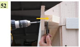
Fasten the trim board with 1 1/4" screw into rake block.
