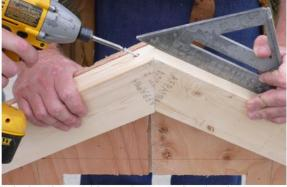
Placing the 2 gable sections together (as shown above), make sure it is square, and then fasten using  $2 \ 1/2$ " screws.
