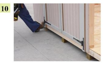
Door panel will attach just as a wall panel, apply pressure on the outside and fasten with 2 1/2" screws on the inside.
