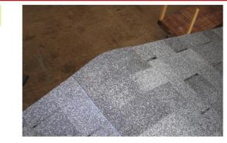
Continue to edge of the building. You can finish with a smaller cap with an adhesion strip.
