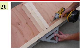
Next you can fasten the bottom of the gable with 2 1/2" screws.
