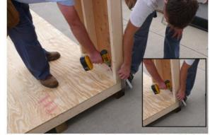
Locate the first wall panel, then set in place. Make sure the wall is flush with the edge of the floor structure, by using an angle. Apply pressure from the outside and secure the wall panel to the floor using  $2 \ 1/2^{\circ\circ}$  screw.
