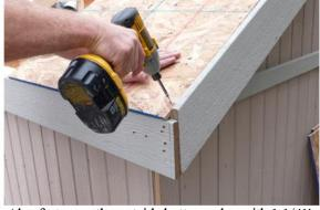
Also fasten on the outside bottom edge with 1 1/4" screws.
