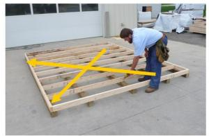
Now place 2x4's, 16'' on center, on top of the 4x4's, place 2 1/2'' screws in each of the 4 corners. Measure from corner to corner to make sure it is square. Now you can fasten each 2x4 to the 4x4's with 2 1/2'' screws.
