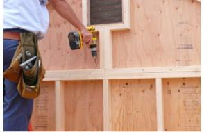
The gable can now be fastened to the top of the wall with 2 1/2'' screws.
