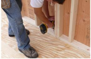
...to completely secure the wall panel to the floor place 2 1/2'' screws 16'' on center
