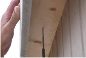
Then fasten from the bottom as well. Secure from bottom of 2x8 top plate with  $2 \frac{1}{2}$  screws.
