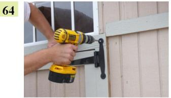
The piece of trim at the top of the double doors will fit behind the door hinge, you will then fasten the trim with a 2 1/2" black headed screw into the hinge through the trim.
