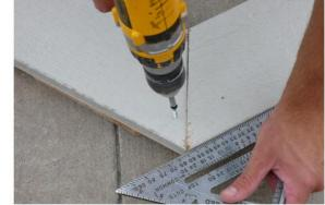
Square peak of 1x6 trim for Rake and fasten onto 2x4 Rake with 1 1/4" screws.
