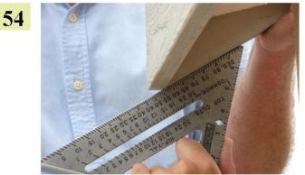
Install outside rake and use angle to make flush with bottom of Fascia.
