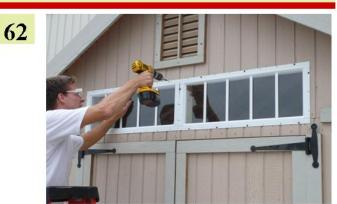
...secure with 3 screws at the top and 3 screws at the bottom, per section.
