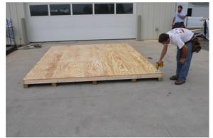
Next set sheet in place and make sure sheeting is flush on both sides. Secure in place by driving 1 1/4" screws through the sheeting into the 2x4s every 8".
