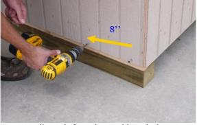
Fasten wall panels from the outside at the bottom with  $1 \ 1/4$ " screws every 8".
