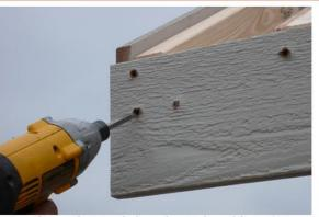
Now fasten the Fascia board to Rake with 1 1/4" screws
