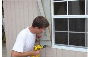
Fasten shutters with 2 1/2" screws in each corner and one in the middle on inside corner.
