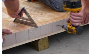
Place the small piece of duratemp siding (this is the piece we set aside to use underneath of the door) below door opening and use angle to make flush. Fasten with 1 1/4" screws approximately 8" on center.
