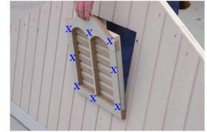
Next install the wooden vent and secure with 1 1/4" screws at each X.
