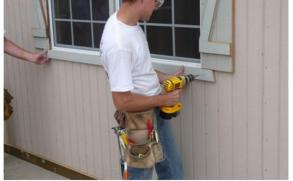
Install trim on the bottom of windows and fasten with  $1 \frac{1}{4}$ , screws.
