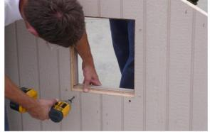
...place 1 1/4" screws in each corner and in the middle to secure the frame.
