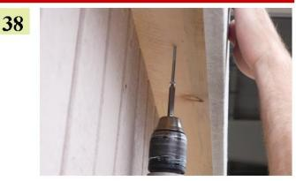
Temporarily fasten the brace to the top plate with a 2 1/2" screw from the outside of the building.
