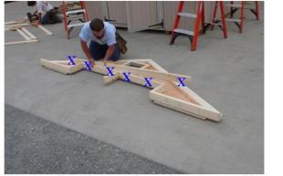
Now install 2x4 brace as shown above, secure with  $2 \frac{1}{2}$  screws on the X's. Then install gable vent as shown in previous pictures. (refer to  $\frac{#21-#23}{2}$ )
