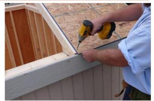
Now you are ready to install the roof sheeting. Start with the bottom sheets. You will fasten each sheet on the outside edge with  $1 \frac{1}{4}$  screws.
