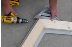
To construct the Rake begin by squaring the rake and fasten with 2 1/2° screws.
