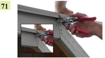
As you secure the drip edge, you will need to snip the drip edge to allow bend along the ridge.
