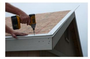
Next your are going to install the drip edge. This will be fasten with 1 1/4" screws.
