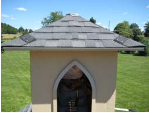
Roof is on top of the Cupola.
