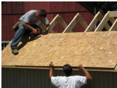
Install next piece and secure with 1 1/4" screws.
