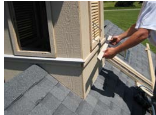
Install Cupola trim as shown and secure with 1 1/4" screws.
