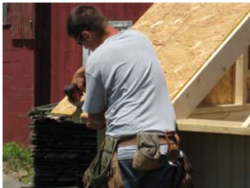
Make sure sheathing reveals are the same on the bottom.
