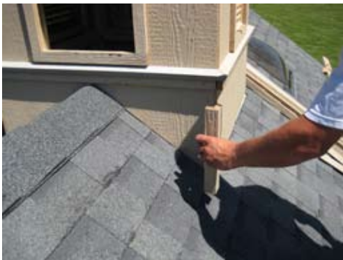
Continue with corner trim. Secure with 1 1/4" screws.
