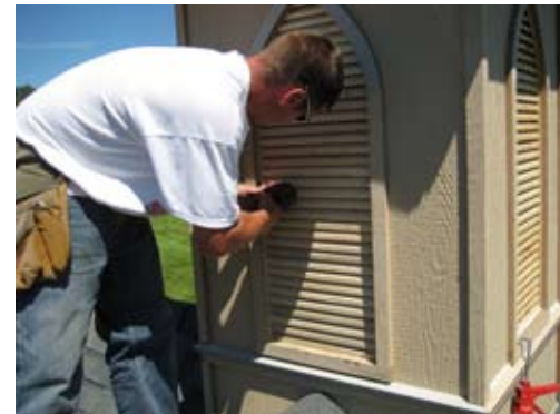
Insert 1 1/4" screws on each side.
