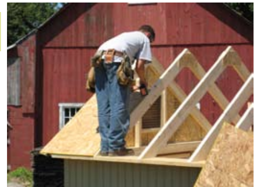
Continue with sheathing.
