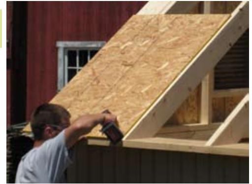
Install first piece of sheathing as shown and secure with 1 1/4" screws.
