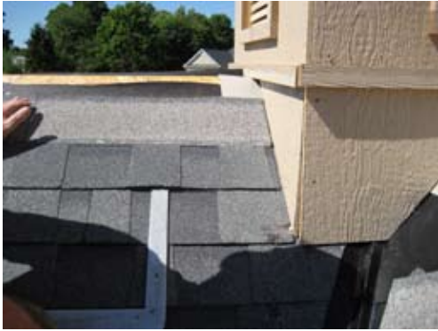
Cupola will be installed after roof is shingled.
