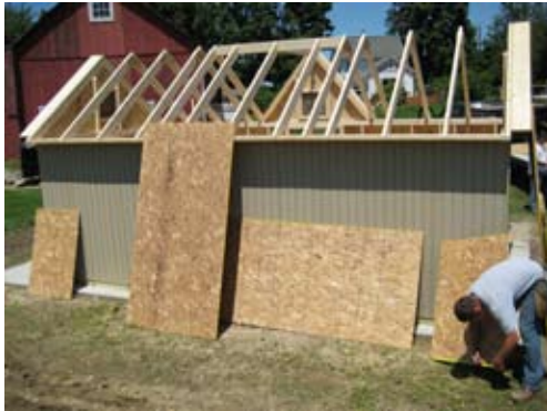
Locate sheathing layout.
