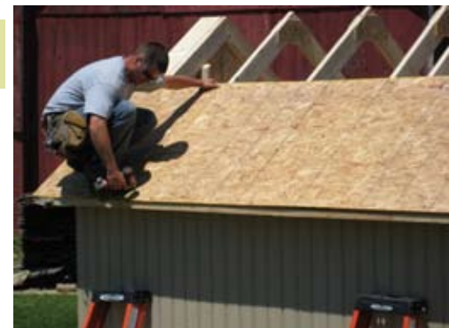
Next fasten bottom corner with 1 1/4" screw as shown.
