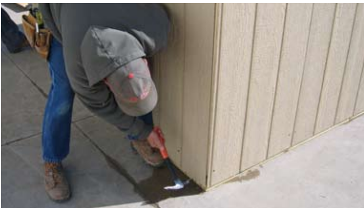
70. Fasten the bottom with 2" nails every 8 inches.
