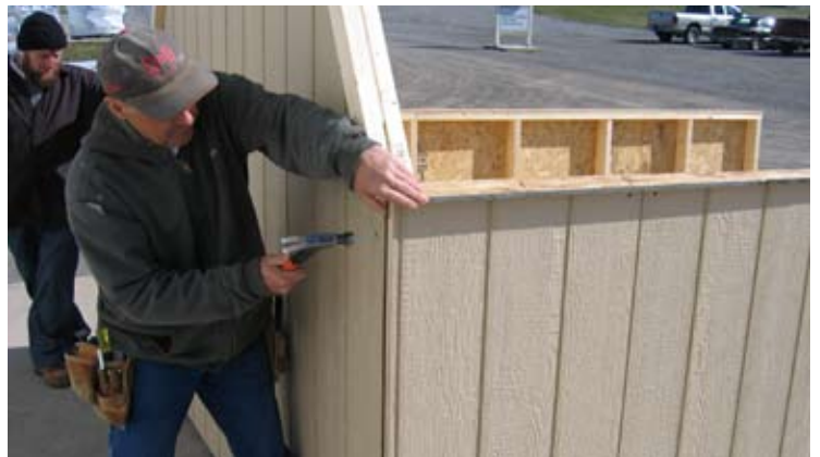
69. Make sure the walls fit nice and tight and fasten with 2" nails every 8".
