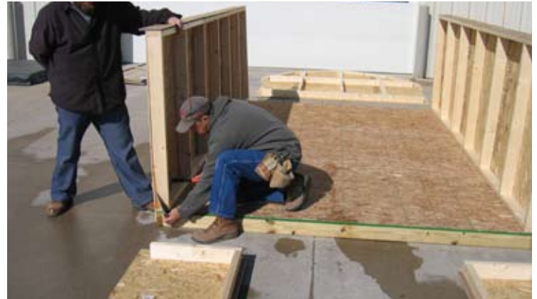
67. Continue with walls.
