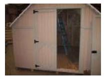
Place spacer bar as shown and install the door using this for a guide. Left side has already been hung.
