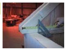
Measure in from the sides and center this. It should measure 5 1/2" as shown.
