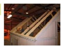
Install trusses in premarked spots. You may have to pull them to the correct position. This is from not fastening the scabs correctly, or from a bowing wall or other factors.
