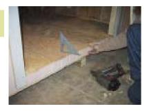
Install 2 small pieces of siding beneath the door. Keep even with the floor.
