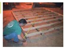
Measure from side to side either way until the measurements are the same. You will then know the floor is square.
