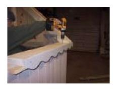
Install the shorter 2x6 with trim. Match the sets with X's and O's on the bottom.
