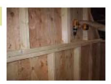
Once it is centered fasten. Be sure to put plenty of screws around the splices.
