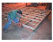
Then place the 4x4 pressure treated runners underneath this frame. Fasten only on the ends.
