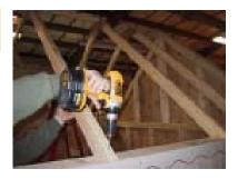
Now fasten the rear truss onto the 2x6. It should be centered between the two trusses.
