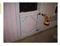
Place door on the spacer bar. Fasten using only one screw per hinge. This way if you need to make adjustments you will not have to undo all the screws.
