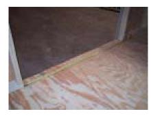
Now install section K. The door opening should measure 54". This is very important. otherwise the door will not fit correctly. You may have to move the panels and possibly the back and front walls to get this measurement.
