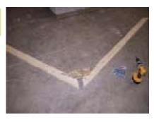
Put the truss angles together. Note: you will have to match the correct angles that match the truss scabs.
