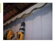
Once the last piece is in place, fasten the blocks underneath to the other piece. This will make the wall and the 2x6's sturdy. Repeat the steps on the other side.
