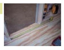
When installing panel C, make sure the door measures 20" from edge to edge then fasten.
