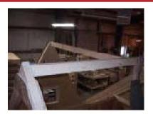
Slide the T-bar piece on top of the dormer, and in between the trusses.
