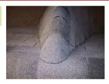
Cut a ridge cap with a rounded edge as pictured and install.
