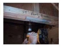
Install the piece of trim as shown on the top of the door frame.
