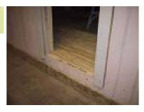
Place spacer bar by edge to use as a guide for door installation.
