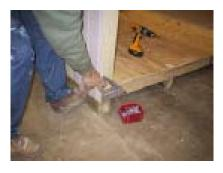
Install section A, keep even with the edge of the floor and push it in against the floor from the outside.
