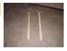
Pictured are the V- channel roof braces.
