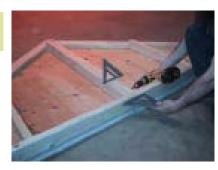
Now fasten panels H and I to each other. Make sure they are even on the bottom. This piece may bow slightly; this can be made striaght in the following steps.
