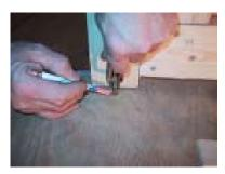
Close the door and mark around the door latches top and bottom.
