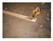
Now fasten the truss scabs, keep the top even. Install one scab on either side of the truss. Make sure the scab does not stick out past the truss.
