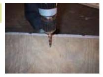
Use 5/16 bit to drill holes for the door latches to slide into.
