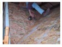
Then fasten the V-braces using black headed screws.
