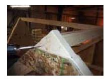
Center the T-bar on the trusses and fasten on both sides.
