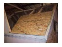
Install the front dormer piece. You should be able to "eye" how it shoots into the corner of the T-bar.
