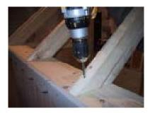
Note, where to place the edge of the trusses. Place on the edge of a 2x6 and not on the trim.
