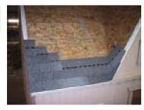
Install the drip edge. Cut tabs off of the shingles and install a starter strip. Notice the glue strips toward the bottom. Fasten with 3/4" roofing nails.
