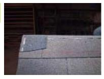
Cut pieces for the ridge cap. See instructions on the shingle package. A regular utility knife works well for this, cut shingles from the back side. To start by cutting one into a smaller piece as shown. Then install on top using 7/8" roofing nails.
