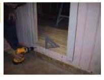
Install a small piece of siding beneath the door. Keep even with floor.
