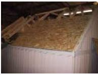
Install sheeting on the back side first. It is very important that the rear truss is in the center of the building. There will be a gap between the OSB and the 2x2 with trim fastened to it. The OSB should run along the edge of the endwall truss and be in the center of the rear truss.
