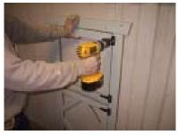
Next install the top door piece. try to center the door between the top trim piece and the bottom door. If both doors work well, install the rest of the screws and remove the spacer bar.
