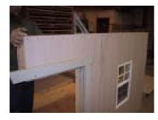
Install section B header block. Be sure to keep even on the top.
