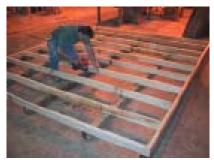
After you have squared the floor, fasten the rest of the 2x4's to the 4x4's.
