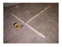
Fasten two pieces together to form a T-bar. Use the premarked center to make sure it is centered. Make sure to use the correct pieces.
