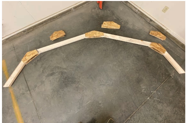
46. Once the truss is assembled on one side flip it over in order to attach the OSB gussets on the opposite side, using 2" nails.
