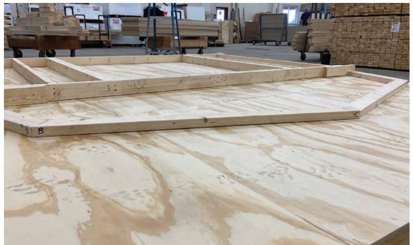
23. Match up trusses parts to the corresponding letters A, B, and C. These will need to be turned the correct way or they won't fit correctly. Fasten using 3" nails.
