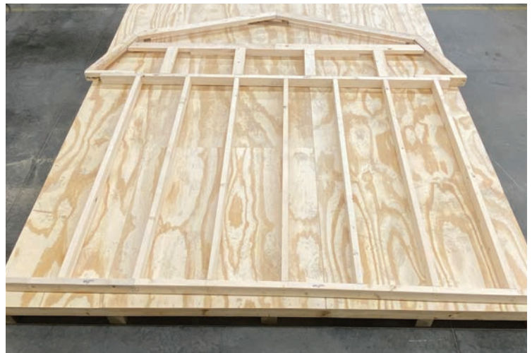
39. Completed back gable wall framing.
