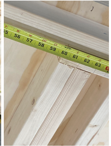
20. Attach a temporary support to the lower part of the door gap in the frame. Ensure the gap's width is correct - it's 48" for a 8' wide unit and 60" for 10' and 12" wide units.
