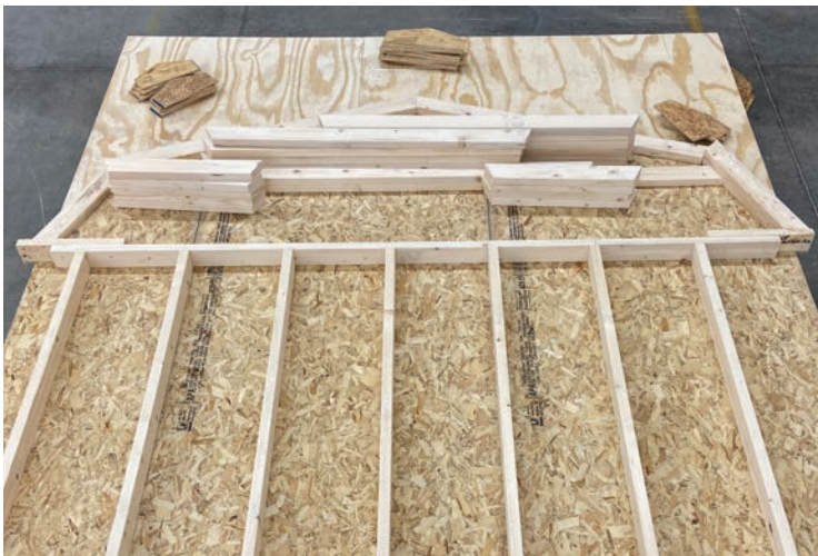
44. Truss Assembly: Locate all the truss parts.
