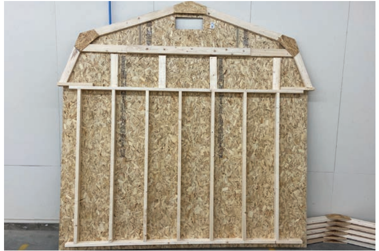
43. Completed gable back wall - interior
