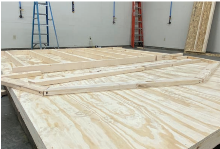
38. Following the WALL LAYOUT DIAGRAM. Put together the top of the back end wall in the same manner as you did previously for the top front end wall. Follow the truss markings A, B, & C.
