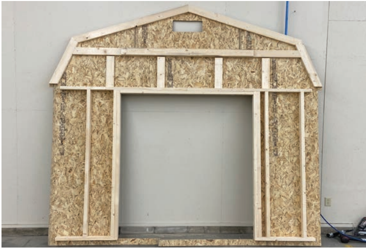
36. Finished Interior Side of Gable Door Wall.
