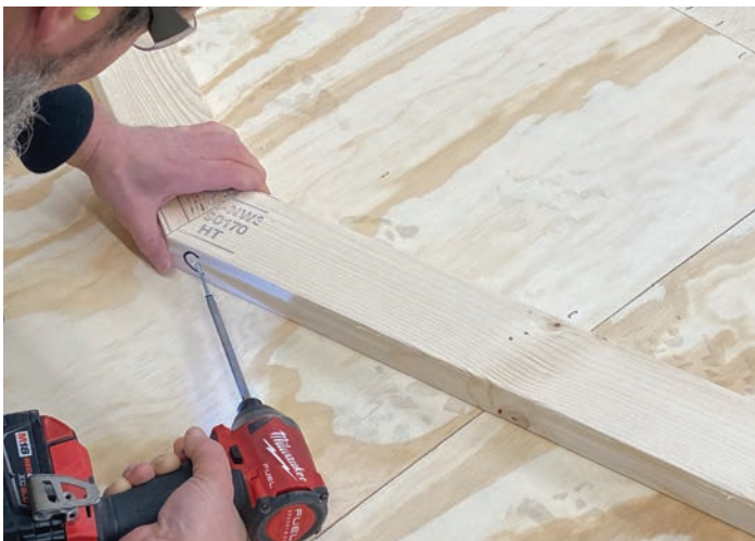
23. Match up trusses parts to the corresponding letters A, B, and C. These will need to be turned the correct way or they won't fit correctly. Fasten using 3" nails.
