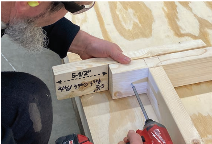
21. Attach the temporary 20" long 2x4 block to the top plate, measure 5-1/2" from the plate's edge as shown, secure with screws, and do the same on the opposite side.
