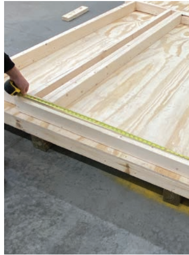
20. Attach a temporary support to the lower part of the door gap in the frame. Ensure the gap's width is correct - it's 48" for a 8' wide unit and 60" for 10' and 12" wide units.
