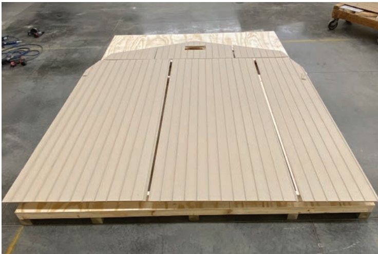
40. Following your SMARTSIDE SIDING LAYOUT DIAGRAM place the siding into position using the same measurements as Steps 30 and 31.
