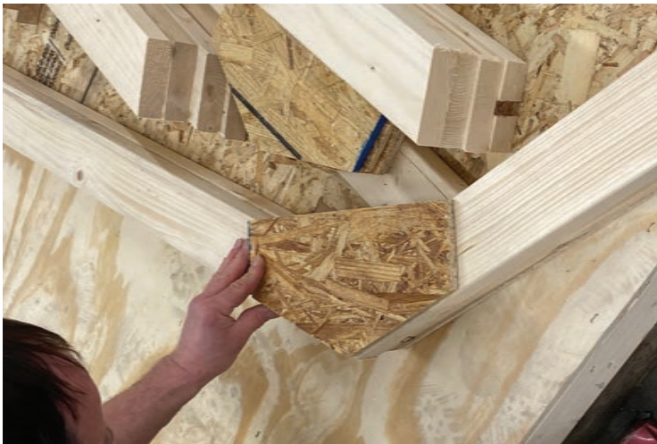
45. Layout OSB gussets, as shown, and secure with 2" nails to start the truss assembly. There are 3 per side.
