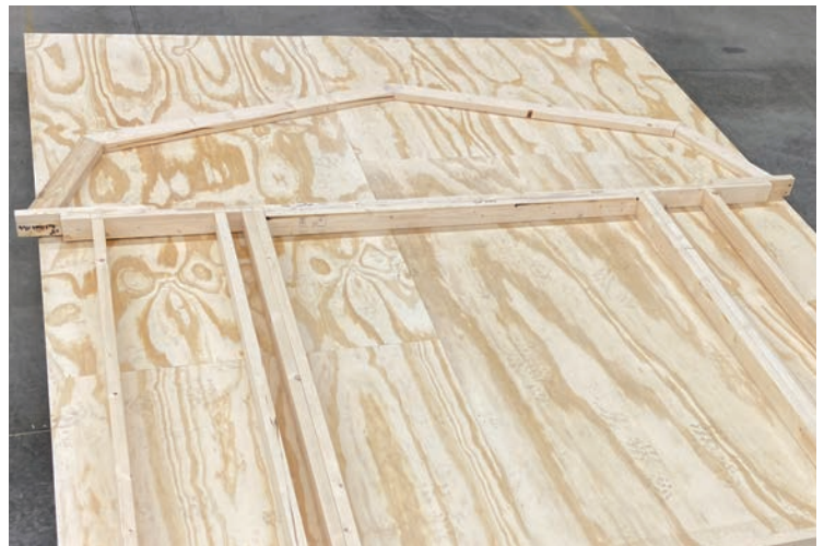
22. Next, Using the WALL LAYOUT DIAGRAM sheet locate the truss pieces for the top of the Door Wall.
