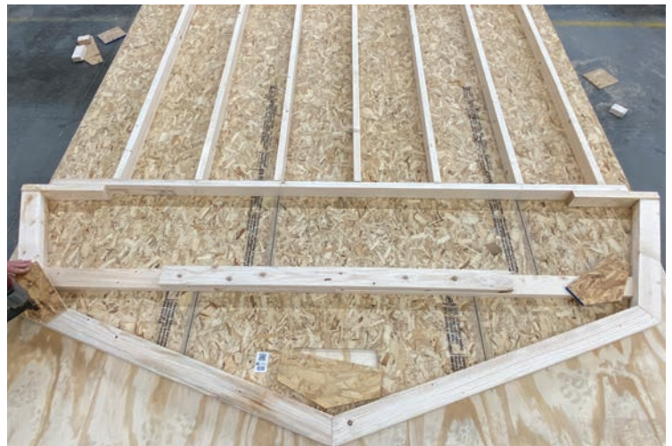
45. You will use the previously assembled gable truss as a template to assemble the trusses.
