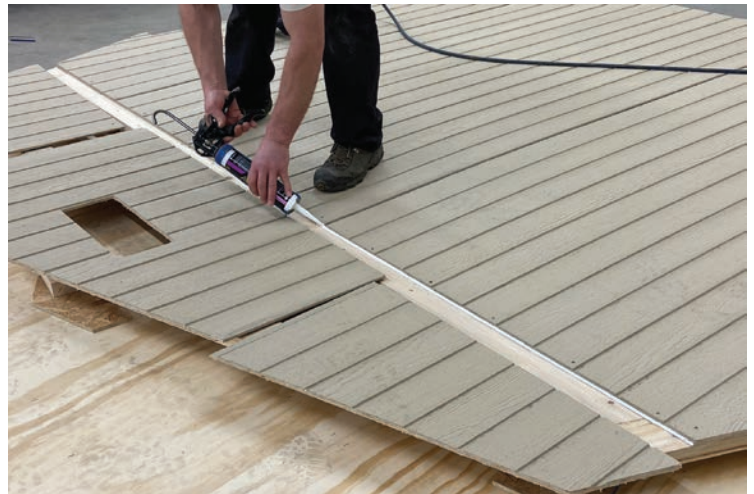
41. Following your SMARTSIDE SIDING LAYOUT DIAGRAM place the small pieces of siding at the top of the back end wall. Optional caulking is recommended. Fasten paneling with 2" nails.
