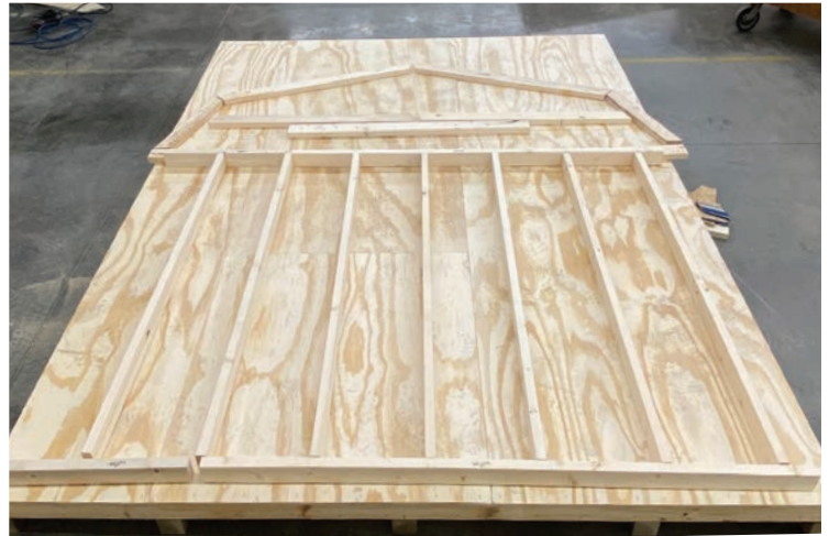
37. Next following your WALL LAYOUT DIAGRAM, layout the framing for the back end wall. Fasten together using 3" nails.
