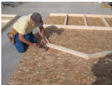
See diagram to match truss A,B, and C. Secure with 3" nails.
