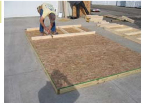
Secure with 3" nails as shown.
