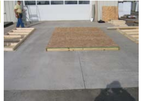
Lay wall to the side as shown.
