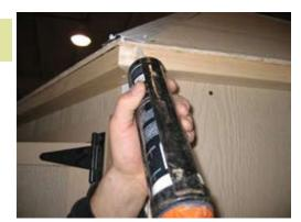
Insert a bead of caulk on the bottom edge of roof panel on all 6 sides as shown.
