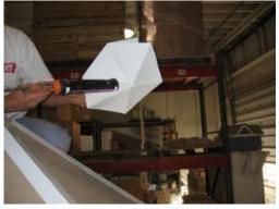
Next locate metal cap for peak and put on a bead of caulk.
