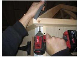
Use angle square and make sure rafter is flush with outside edge of 2x6 top plate as shown.
