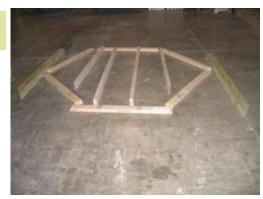
You will have 6 pieces for the rim, which are cut on an angle at both ends. (4) 2x4 joists and (2) 4x4 runners
