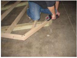
Continue with 2 1/2" screws securing 2x4 Floor into 4x4 runners.
