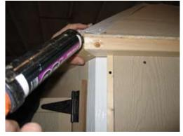
Insert a bead of caulk on the bottom edge of the ridge as shown to keep moisture out.
