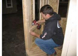
Remove 2x4 from door on the inside as shown.
