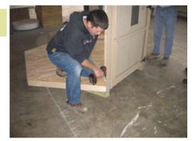
Secure with 2 1/2" screws on each corner.
