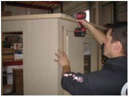
To secure top plates fasten with 2 1/2" screws into 2x6 top plate.
