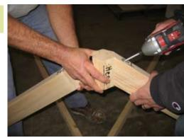
The rafters are marked top and bottom. Make sure top is up and secure with 1 1/2" screw as shown.
