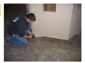
Fasten bottom into the floor with 1 1/4" screws every 8 " to 10".
