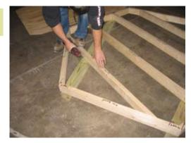
Once all corners measure the same, Fasten the rest of 2x4 joist into 4x4's as shown with  $2 \frac{1}{2}$ " screws.
