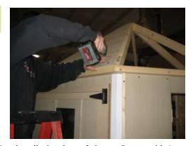
Next install triangle roof pieces. Secure with 1 1/4" screws.
