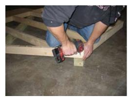
Secure with (2) 2 1/2" screws on each side.
