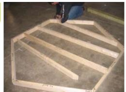
Next install joist as shown. Rims are marked for joist placement. Secure with (2) 2 1/2" screws on each end.
