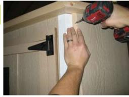
Next install small wood strip on top of aluminum trim with 1 1/4" screws.
