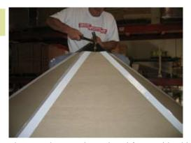
Place metal cap on the peak and fasten with white trim nails as needed.
