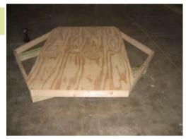
Next locate CDX plywood flooring with angles cut on all corners. Plywood is designed to fit the floor.
