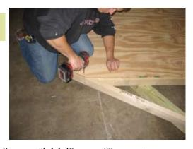
Secure with 1 1/4" screws 8" on cemter.
