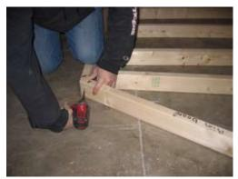
Fasten (6) pieces of rim as shown and secure with 2 1/2" screws (2) per side.
