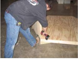
Make sure wall is pushed against the floor before fastening.
