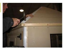
Install Aluminum Ridge and fasten with white finish nail.
