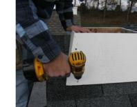
To attach the base to the roof you will want to screw in 1, 2 1/4" screw at an angle into each corner.
