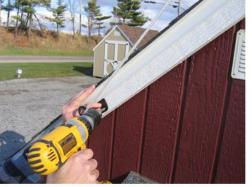
Install the bracket on the side of the trim with 4,  $1 \frac{1}{4}$  block head screws.
