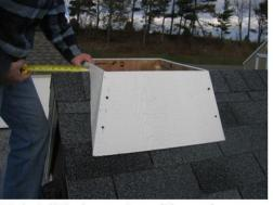
To install the base on top of the roof, you will want to measure 6" from the edge of the roof.
