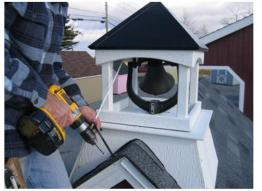
Now install the brackets, which the rope will slide through, on the peak and front edge of the roof. To attach the brackets you will use 4, 2 1/4" screws.
