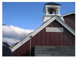
The rope, which is already fastened to the bell, will then slide through the bracket on the roof and again slide through the bracket mounted on the front of the trim.
