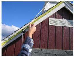
When installing the bracket for the front edge of the roof, measure 29" from peak to bracket.
