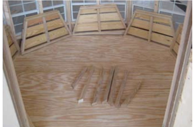
80. Place treated shelves on inside as shown.
