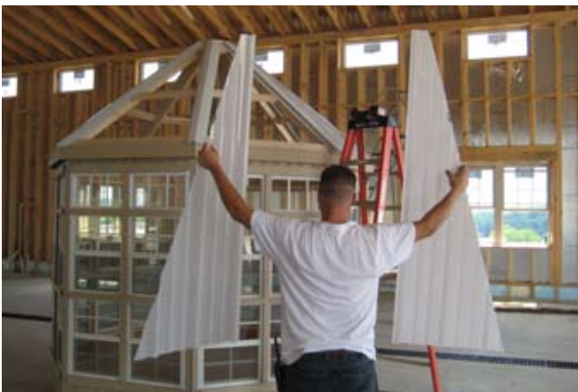
71. Next locate weather-stripping and sunsky roofing.
