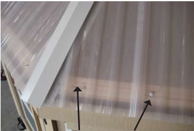
77. Insert screws beside each rip as shown.
