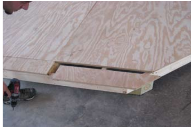
20. Securing the last piece of flooring.
