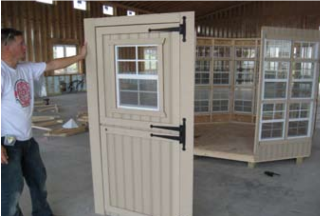
31. Next locate wall with door and install.
