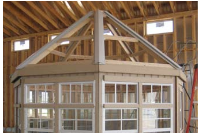
70. Metal corners are done.
