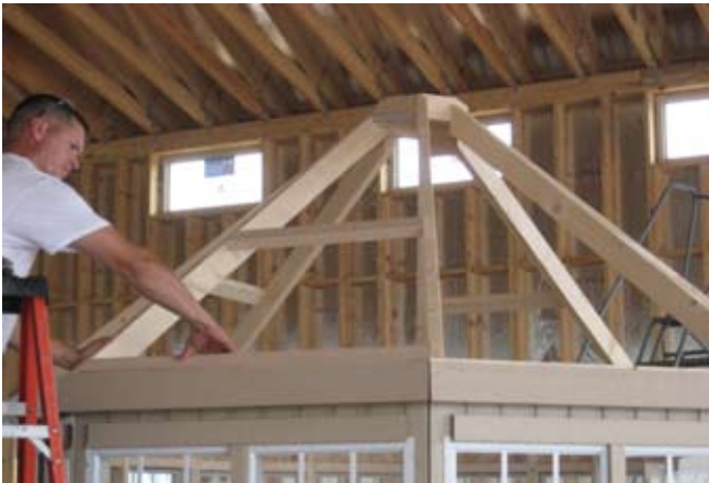
57. Secure bottom of rafters on top plate before doing the top.
