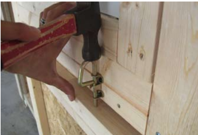
33. Secure with 1 1/4" screws. Use hammer and tap on top of bolt as shown to locate hole to drill.
