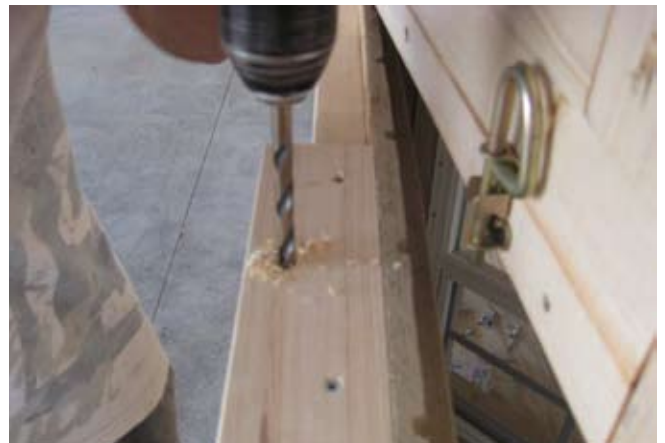
34. Use 3/16" bit and drill hole in bottom of door as shown.
