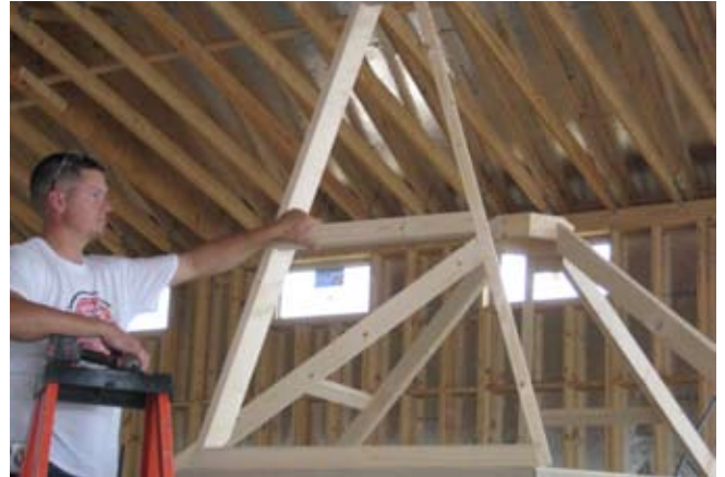
56. Next install last 2 rafters.
