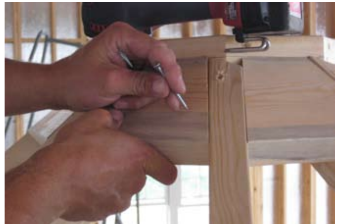
60. Secure blocks with 2 1/2" screws as shown.
