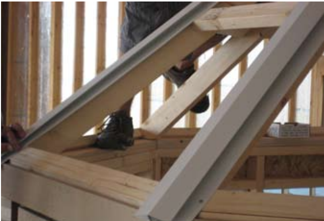
69. Metal corner installed.
