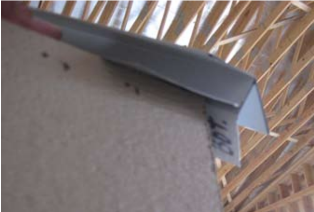
67. Metal corners are marked underneath bottom, so you need to make sure they are on the bottom.
