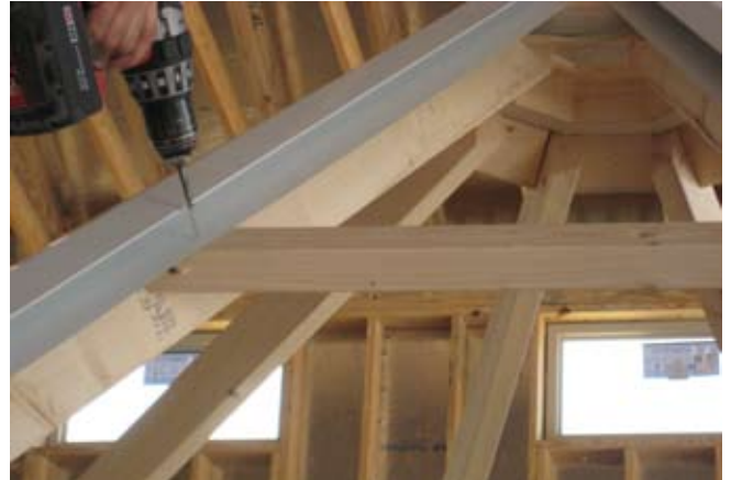
68. Secure with (3) 1 1/4" screws per side.
