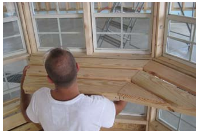
84. Continue installing shelves on 7 walls.
