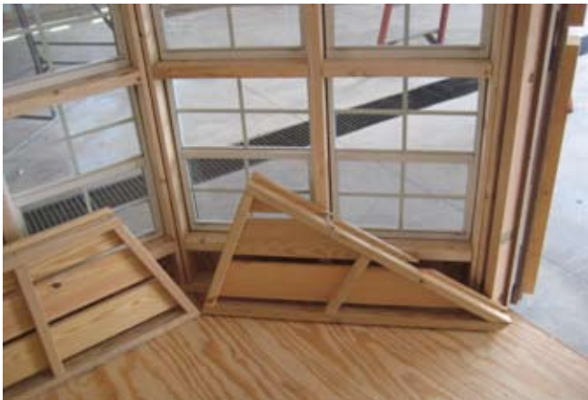
81. Place treated shelves on inside as shown.
