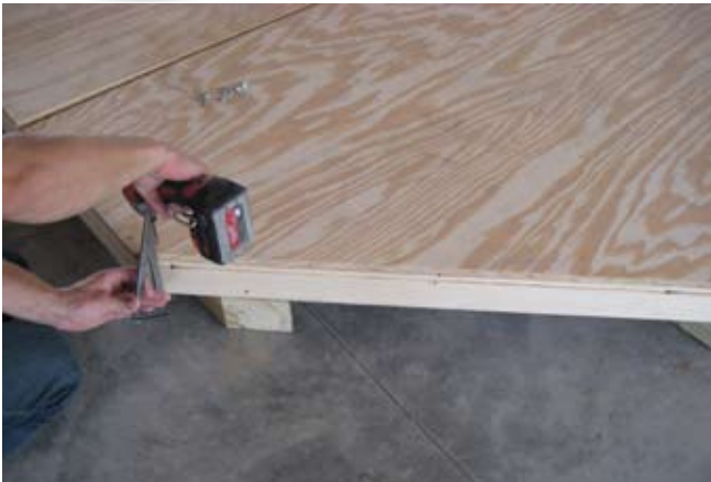
19. Continue with fastening floor. Secure 1 1/4" screw every 8" to 10".
