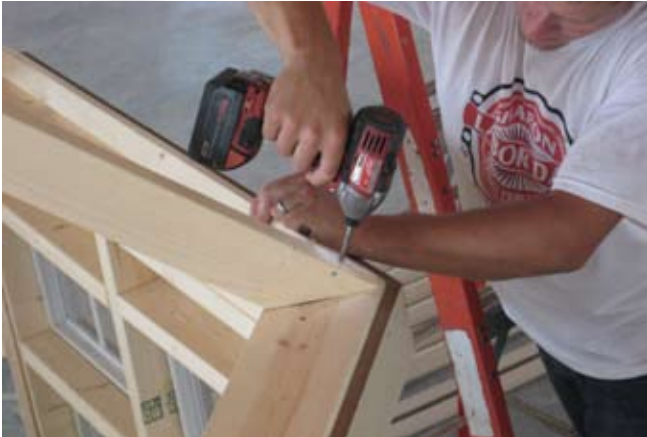
55. Install rafters as shown.
