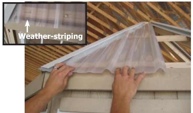
72. Place the weather-stripping under the sunsky roofing. Install the sunsky roofing as shown.
