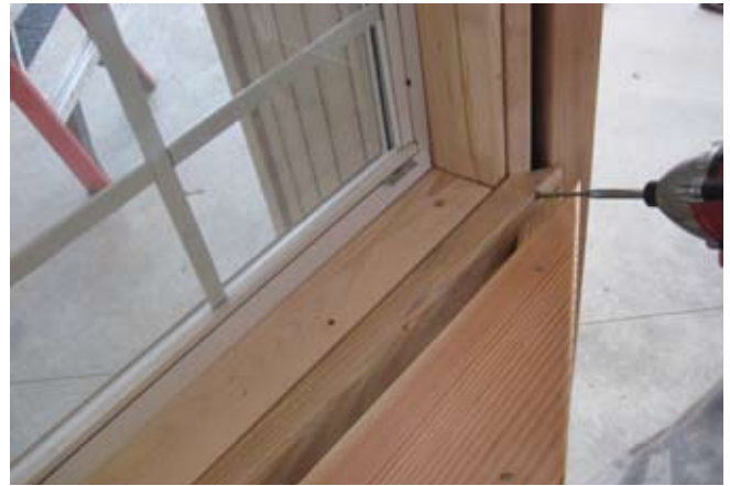
82. Next start installing shelves at corner as shown. Keep flush with top of window sill and secure with 2 1/2" screws. Deck screws are provided for treated shelves.
