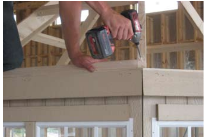
58. Secure rafter with 2 1/2" screws.
