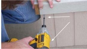
Secure corners of chimney using two (2) 11/4" black headed screws per side.
