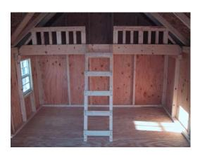
Install the ladder. Put screws in the top and bottom by the floor. Make sure everything is fastened securely before using.
