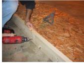
Slide loft pieces together and fasten with screws in front. Make sure loft pieces are tight together or loft may not fit in house.
