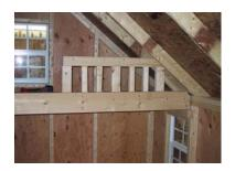
Install left and right railing. Note how it is fastened on the inside of the 2\*6.
