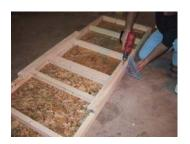
Add a 36" 2\*3 brace to the back Bottom of the loft.
