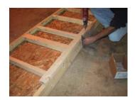
Add a 36" 2\*3 brace to the front bottom of loft. Use plenty of screws.
