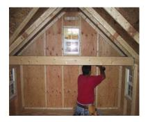
Install the loft bottom or main piece, this slides on top of the loft bottoms. Fasten this with screws. Make sure it is secure.
