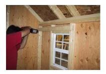
Install the two loft bottoms. This is what the loft will rest on. Install the slanted edge toward the front. From the top of the 2\*3 to the floor it should measure  $42\frac{1}{4}$  inches.
