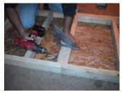
Turn loft around and fasten with screws from either side.
