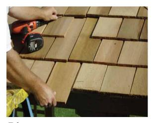
**51.** Roof **Filler Shingles** are included to cover roof seams. Starting at the bottom, slide the first Long shingle in until flush with other bottom shingles.
