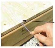
Hint: Use a chalk line to mark location of floor joists to determine screw placement.
