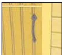
A. Line up Handle with hole. Attach with 3/4" screws.
