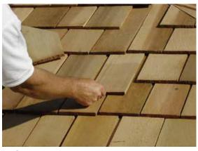
**50.** Slide in another Filler Shingle and attach as per **Step 49.** On your last row of shingles, the filler shingle is precut to fit properly. Attach to roof with 2 finishing nails per shingle.
