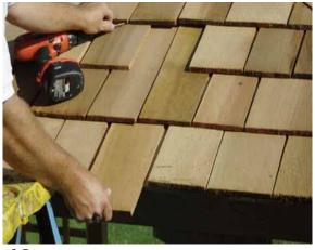
**48.** Roof Filler Shingles are included to cover roof seams. Starting at the bottom, slide the first Long Filler Shingle in until flush with other bottom shingles. See step 49 for proper attachment.
