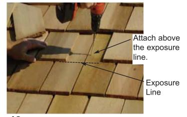
**49.** Screw first filler shingle down to rafters using 1 - 2 1/2" screw per panel (2 in total). Make sure to screw into both rafters.
