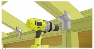
**41.** Attach all **Single** and **Double Rafter Brackets** where rafters meet Top Wall Plates inside of shed. Attach with 2 - 1 1/4" screws and 2 - 2" screws per Single Rafter Bracket and 6 - 2" screws per Double Rafter Bracket.
