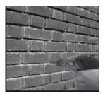
13) After drilling pilot holes or anchor holes (following manufacturers installation instructions), attach head rod clamps to wall ensuring a secure, wobble free connection is made and clamps are level.
