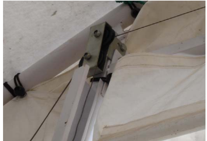
Double Pulley Nearest Winch Assembly
