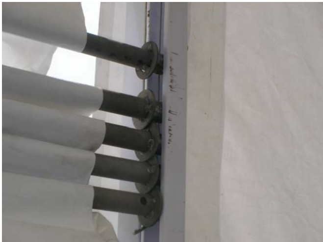
Door Tubes Inserted Into Door Track
